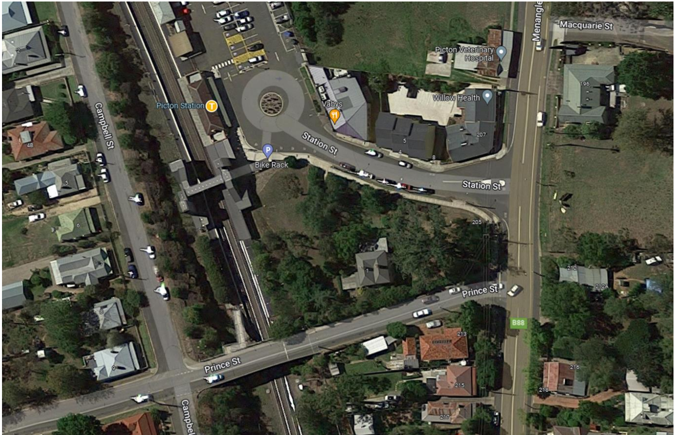
Figure 1: The Prince and Menangle Streets Intersection
