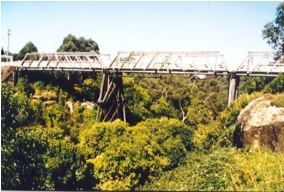
Figure 2: Constructed in 1897 Picton's Victoria Bridge, a timber truss bridge over Stonequarry Creek is still in use today
