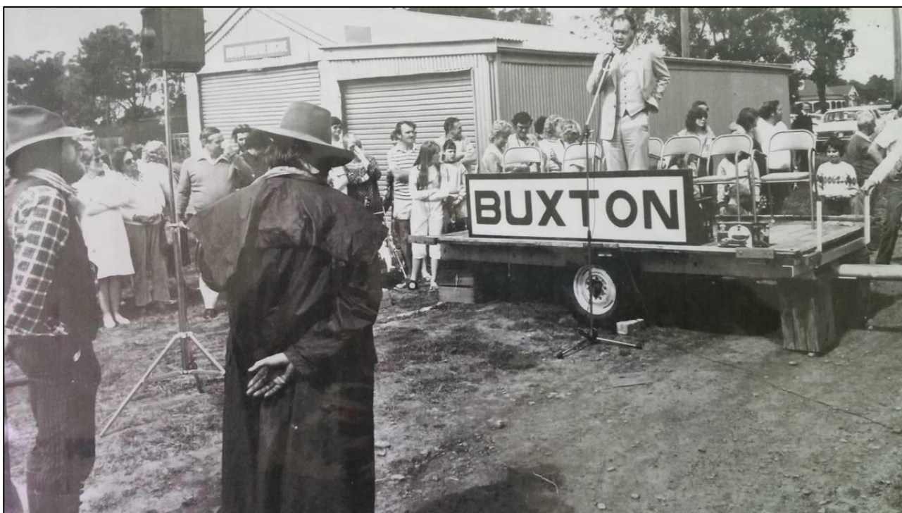
Figure 2-1 Historic photo of Buxton community (Source: Link: https://www.stonequarry.com.au/towns/buxton.html )
