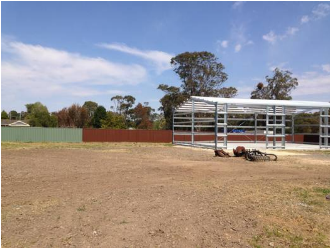
Figure 13 – Newly constructed metal shed on concrete slab footing
