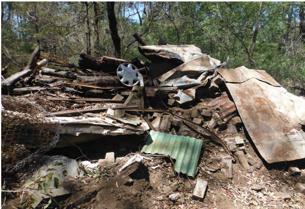
Photo 18 - Stockpile of Building Demolition with ACM fragments (AEC2)
