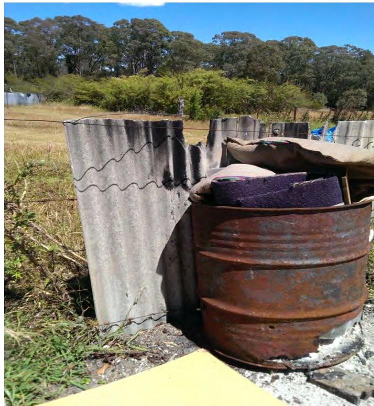
Photo 14 - 44 Gallon drum used as a bomb fire, damaged corrugated asbestos sheeting to the rear. (AEC4)
