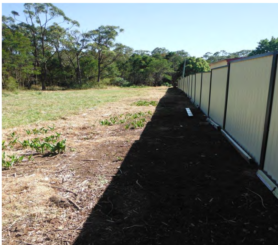
Photo 22 - Newly Constructed Fence with some fly tipping and PACM Fragments on Ground Surface (AEC17)
