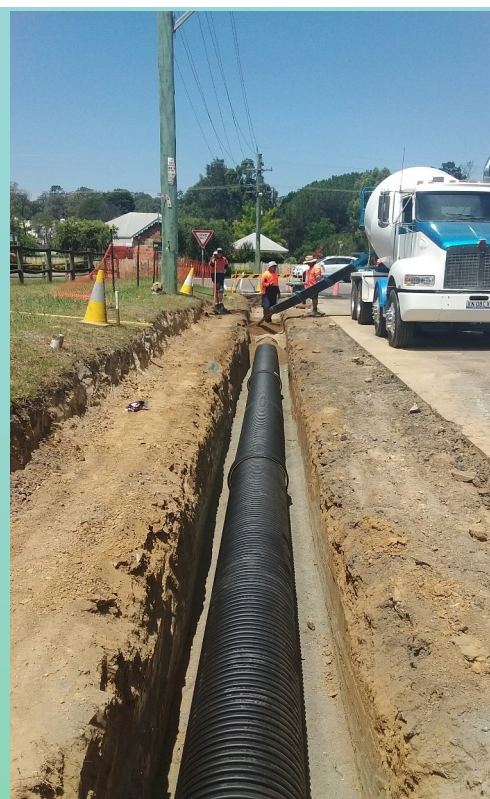
Stage 1 Bridge St, Picton
