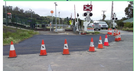
Station St, Douglas Park
