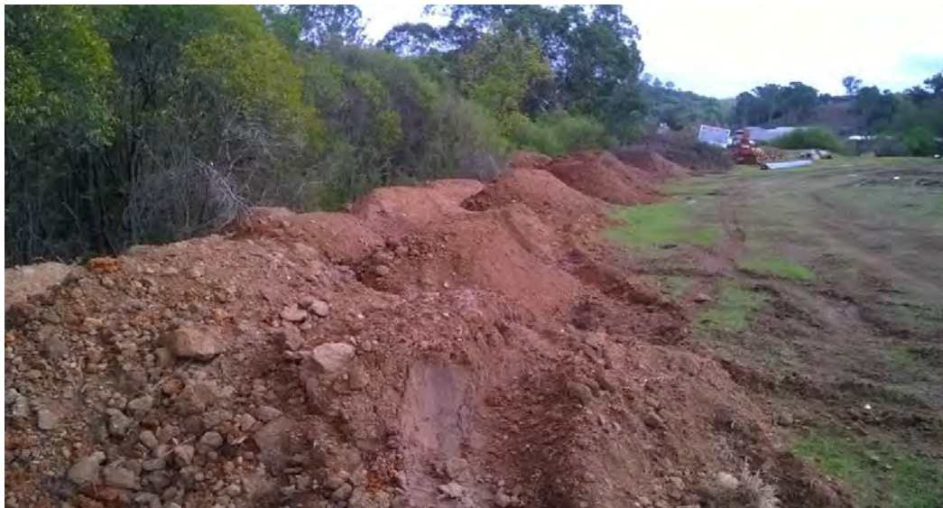
Drawing 4 - Stockpiles of imported orange and brown clay fill (looking west). Photograph taken 2/7/18
