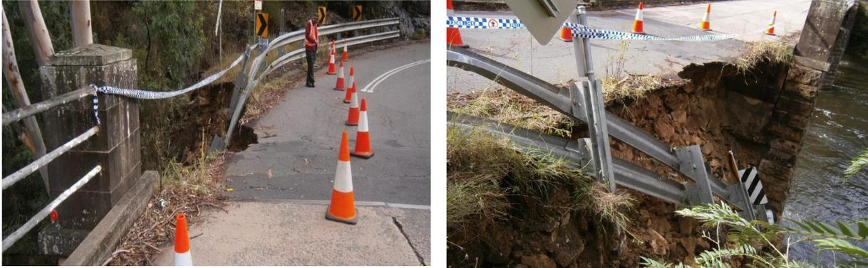
Photos 2 & 3— Extracted from Coffey's Geotechnical Investigation and Concept Design Report, Aug 2016 - View of the failed bridge and retaining wall observed on 6 June 2017.
