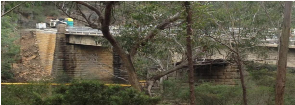
Photo 6 – Repaired wall at Cataract River Bridge, Broughton Pass.
