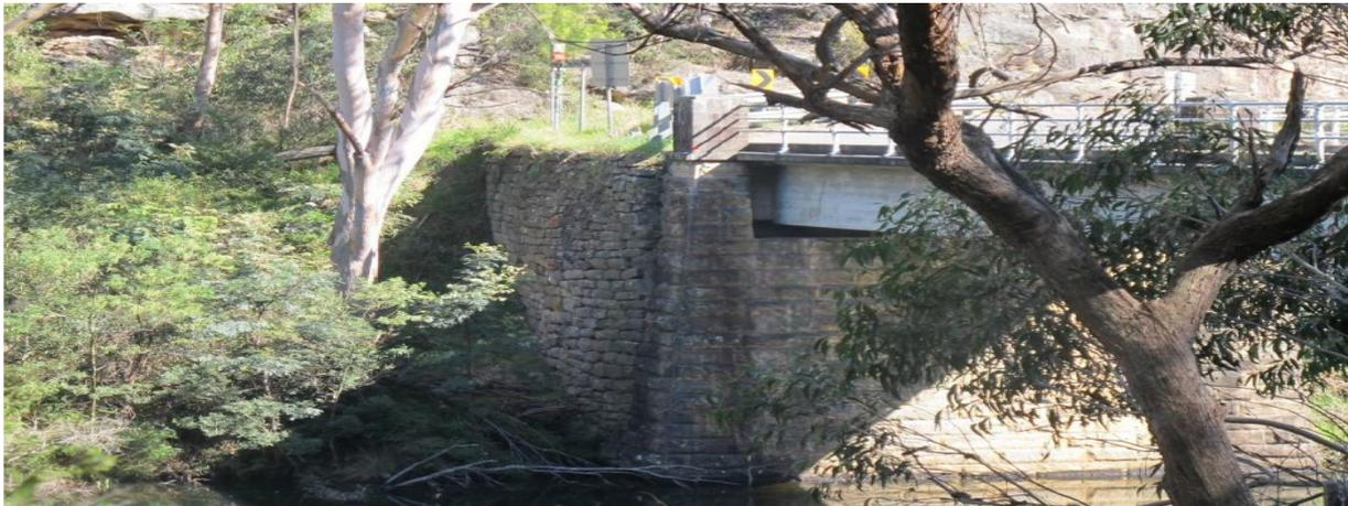
Photo 1 – Extracted from Coffey’s Geotechnical Investigation and Concept Design Report, Aug 2016 - View of the western bridge abutment and dry packed stone wall supporting the road formation on the southern side of the road approach to the bridge, before the damage (Picture taken in September 2011).
