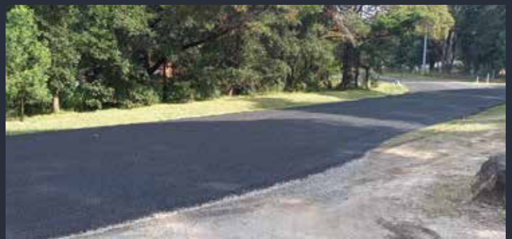
SURFACE SEALING ON BINALONG ROAD TO PREVENT ROAD DETERIORATION
