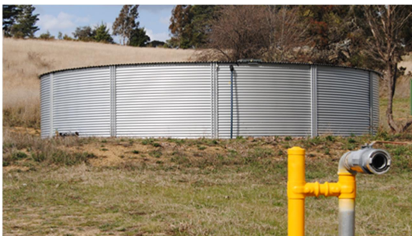
Example of a storz connection associated with a dedicated water storage tank used for dedicated firefighting purposes
