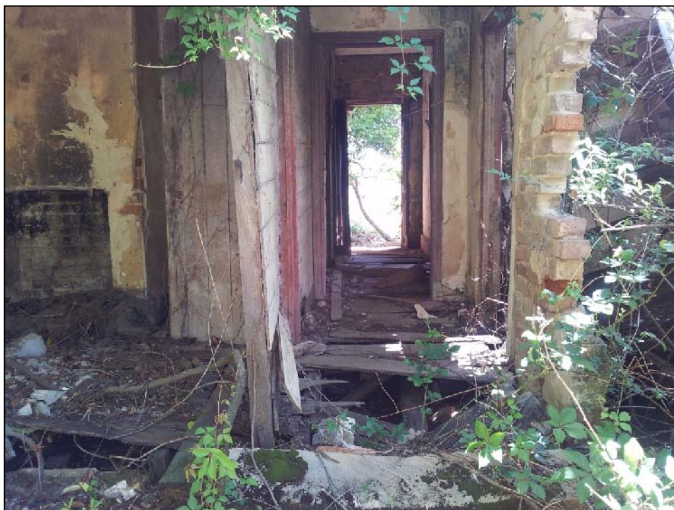
Plate 3: Internal photo of Abbotsford Homestead. Potential for lead paint and asbestos materials.
