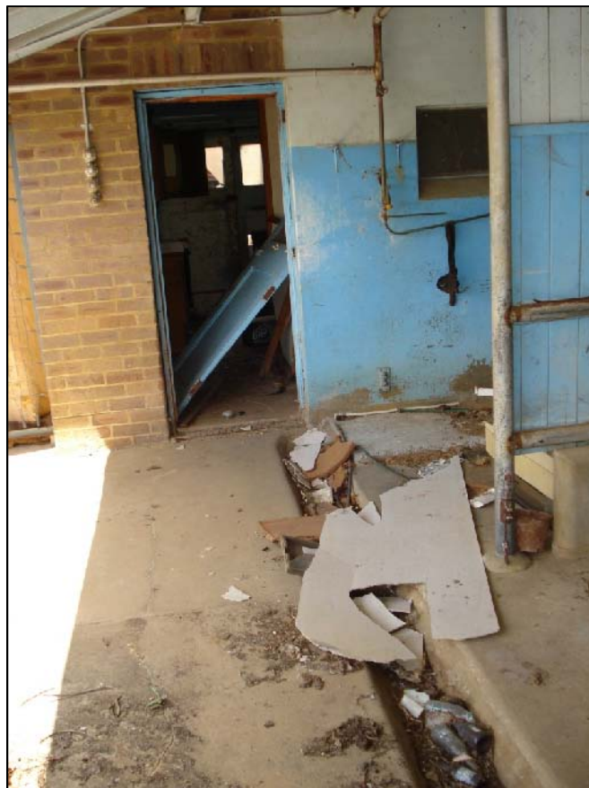
Plate 10: Abandoned milking shed and office. Asbestos sheeting and fragments everywhere..
