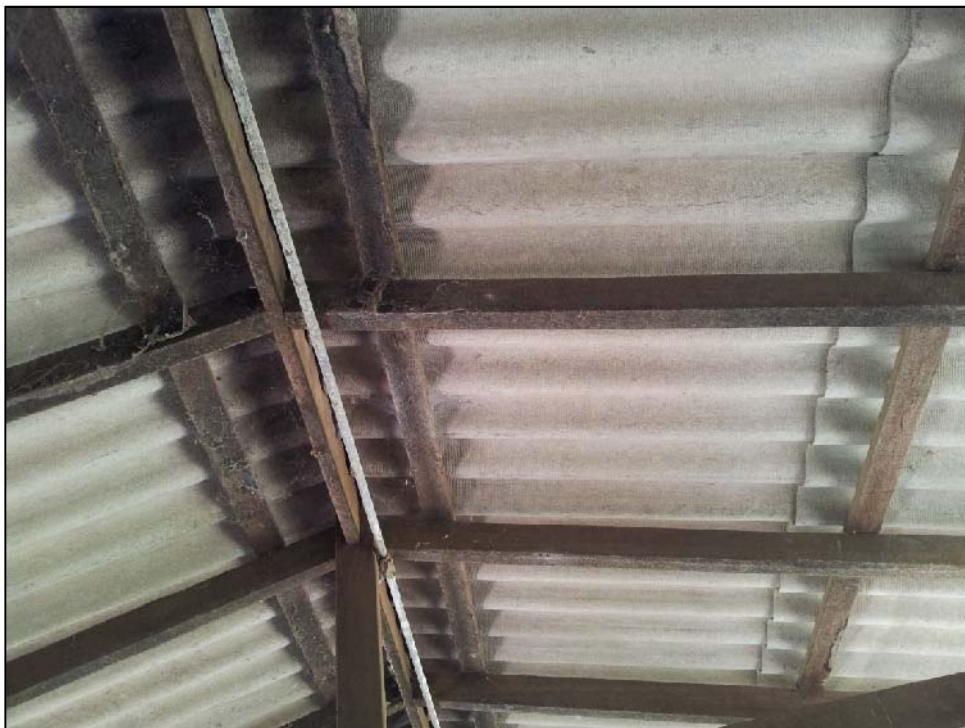
Plate 24: As above with close-up of asbestos roof.
