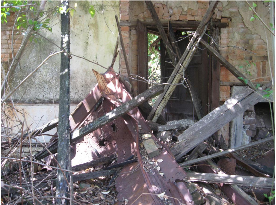
Figure 19 — view inside the ruined homestead showing the only remaining door of six panels with some architrave timbers remaining. Sandstone blocks can be seen on the right, where the original mantelpiece has been lost. The rusting steel is the remains of the pressed metal ceiling, likely added in the Federation period.
