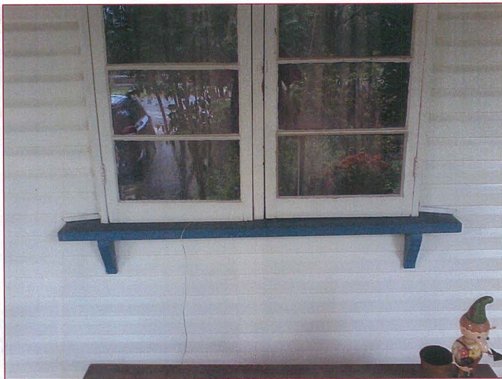
Figure 30: Double casement window and sill, "Yeovil"
