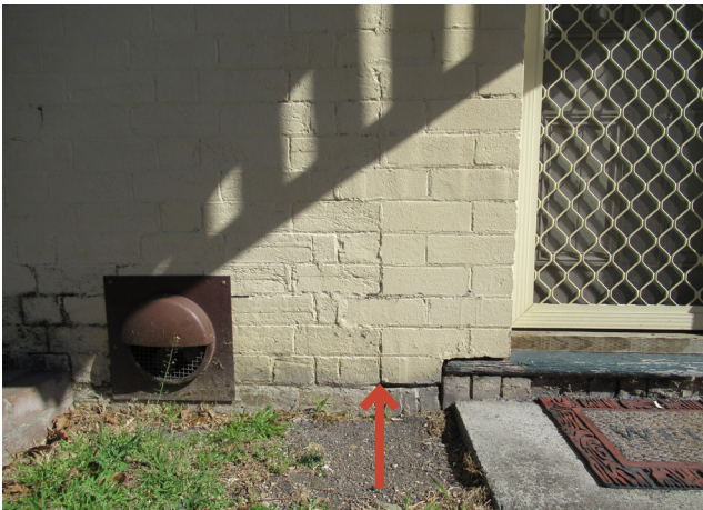
Figure 2.5 Detail of the side (eastern) elevation of the subject building showing the apparent change in brickwork, indicated by a red arrow
