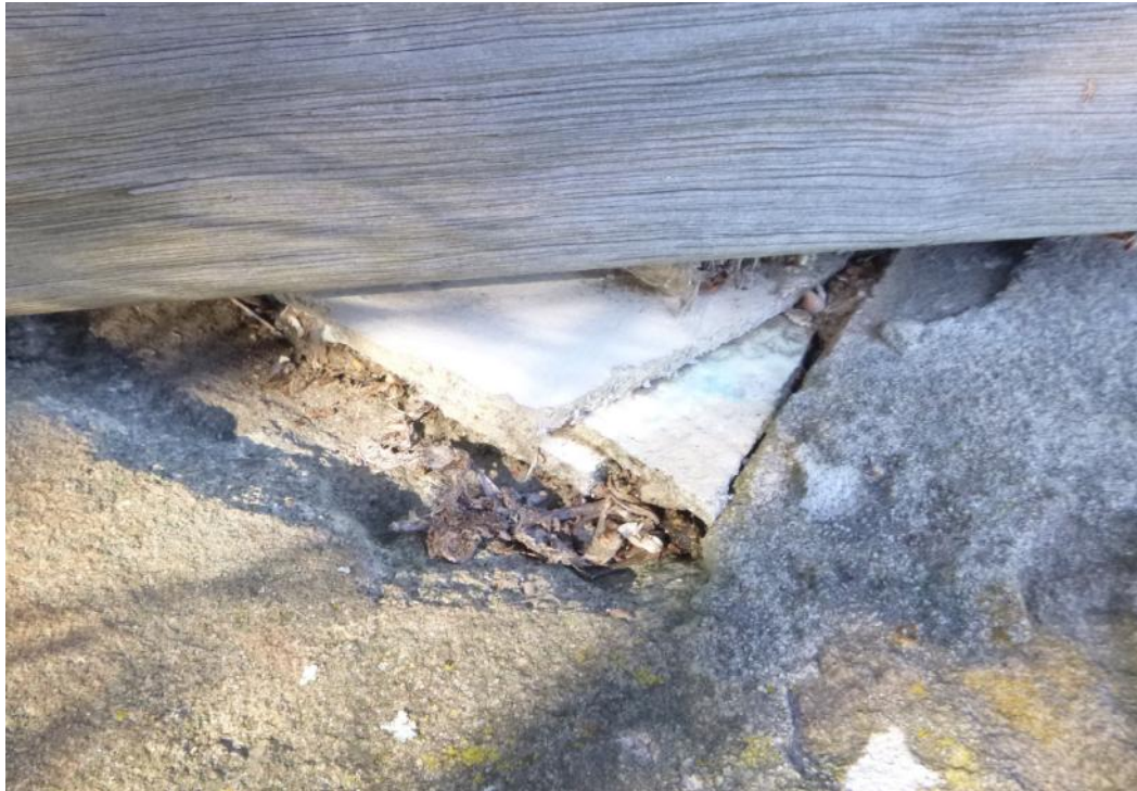
Photograph 3 - Presumed asbestos containing fibre-cement
