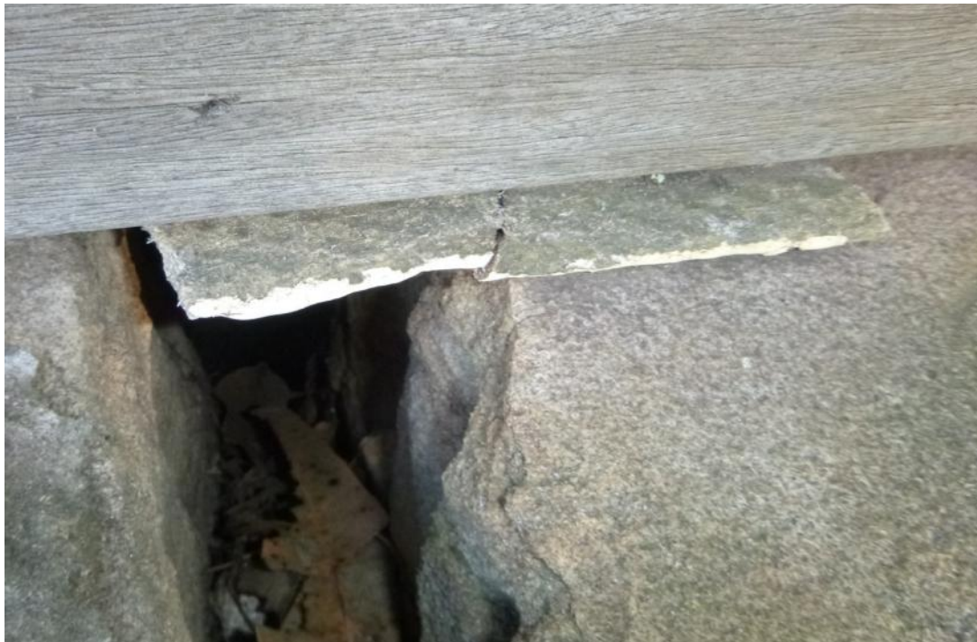
Photograph 2 - Presumed asbestos containing fibre-cement
